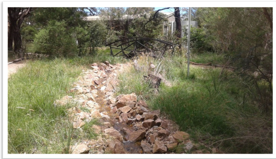
Figure 6. Creek constructed from local stone
